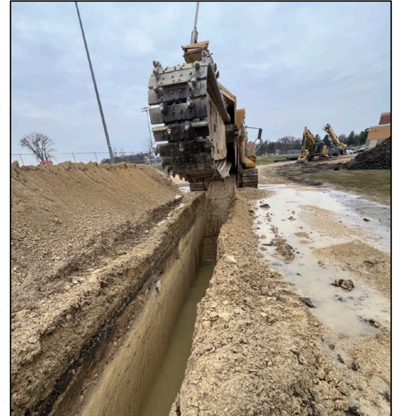
Rock Removal for Site Utility Piping & Structures
